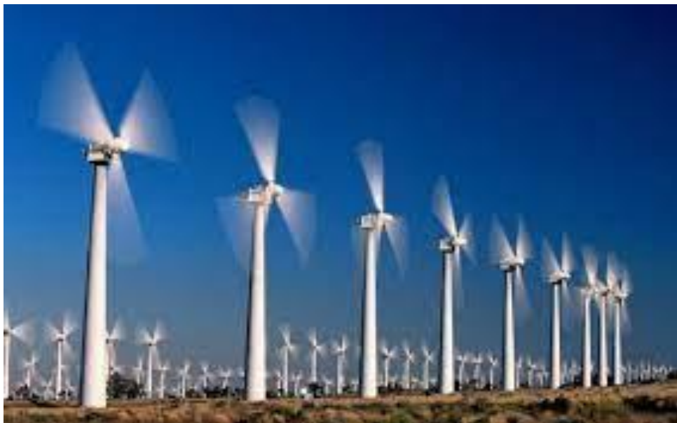
Figure 5 AEDB Wind Power Plant
